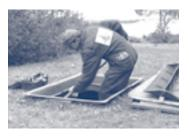
pumped with a regular sewage disposal truck. The replacement filter must be installed by an authorized agent. Easy access to the lid is essential for maintenance purposes.
