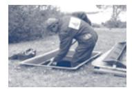
The peat filter must be replaced when it can no longer assure its filtering performances, as determined by one of PT aqua's specialists depending on use and compliance with the above guidelines. The filter bed is easily pumped with a regular sewage disposal truck. The replacement filter must be installed by an authorized agent. Easy access to the lid is essential for maintenance purposes.
