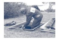
The peat filter must be replaced every eight (8) years at the most, depending on use and compliance with the above guidelines. The filter bed is easily pumped with a regular sewage disposal truck. The replacement filter must be installed by an authorized agent. Easy access to the lid is essential for maintenance purposes.
