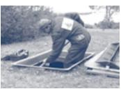
The peat filter must be replaced every eight (8) years at the most, depending on use and compliance with the above guidelines. The filter bed is easily pumped with a regular sewage disposal truck. The replacement filter must be installed by an authorized agent. Easy access to the lid is essential for maintenance purposes.
