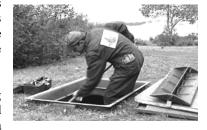
regular sewage disposal truck. The new filtering media must be installed by an authorized agent. Easy access to the lid is essential for maintenance purposes.
