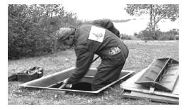
The maintenance of your Ecoflo® Biofilter is carried out by Premier Tech Aqua or an authorized agent. This service includes a visual inspection of all components and verification of operation, as well as maintenance of the filtering media. Easy access to your system's lid is essential for maintenance and for filtering media replacement
