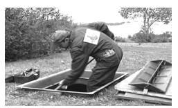
The maintenance of your **Ecoflo<sup>®</sup> Biofilter** is carried out by **Premier Tech Environnement** or an authorized agent. This service includes a visual inspection of all components and verification of operation, as well as maintenance of the filtering media. **Easy access to your system's lid is essential for maintenance and for filtering media replacement purposes.** You will be given a maintenance record after each inspection, which you should keep with this manual in a safe place.
