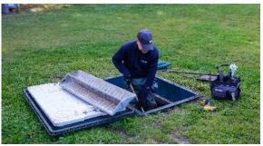
years. However, your ECDn's filtering media must be replaced before the system's treatment capacity and performance begins to deteriorate. The filtering media is easily pumped out using a truck adapted to emptying primary tanks. The new filtering media is then installed by an authorized agent or the pumper.
