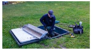
years. However, your ECDn's filtering media must be replaced before the system's treatment capacity and performance begins to deteriorate. The filtering media is easily pumped out using a truck adapted to emptying primary tanks. The new filtering media is then installed by an authorized agent or the pumper.
