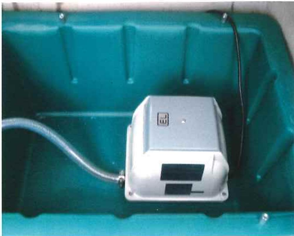
Figure 6: Blower of the ASP 06 with a capacity of 100 l/min.
