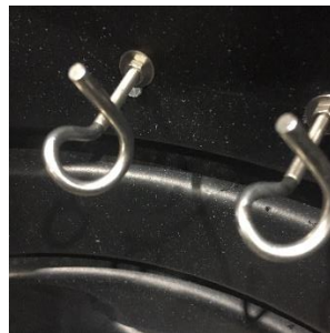
Hang chain onto hooks in manway to aid future access
