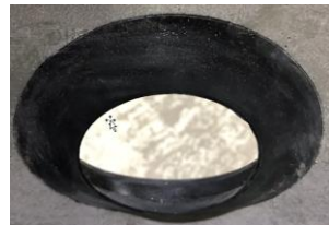
Inside of grommet fitted.
