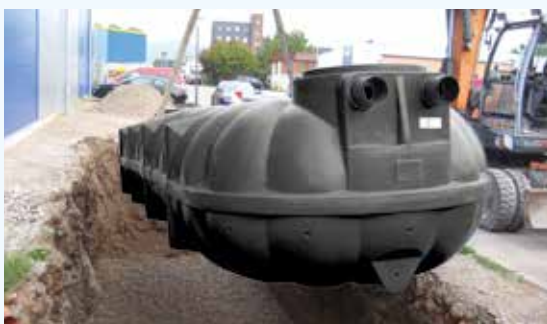
Installation NEO infiltrationstank 10 000 l
