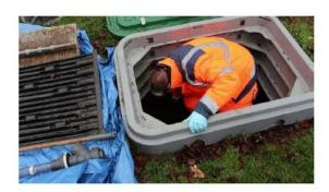
Septic tank should be de-sludged. The emptying of the septic tank must always be carried out by a company specialized in the management of sewage sludge
