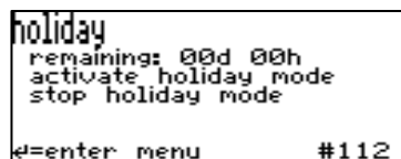
Control Panel Display
