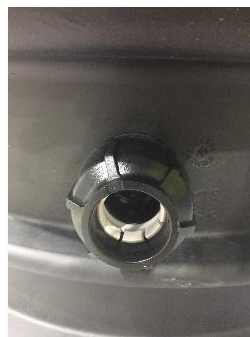
Cut hole in manway to position pump outlet pipe
