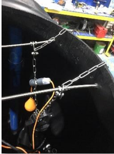
Pump hung on threaded bars
